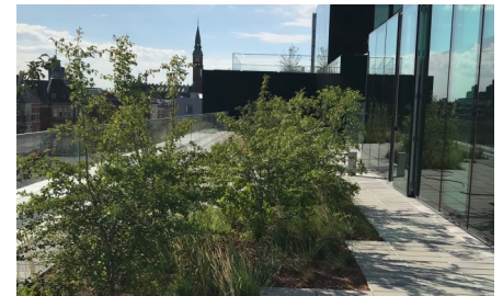
Approx. 3.000 m 2 of walkways and vegetated areas have been installed on various terraces on different building levels.
