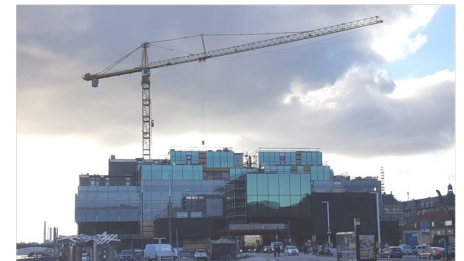
Green Roof logistics were a big challenge: the crane had to be placed on a busy intersection.
